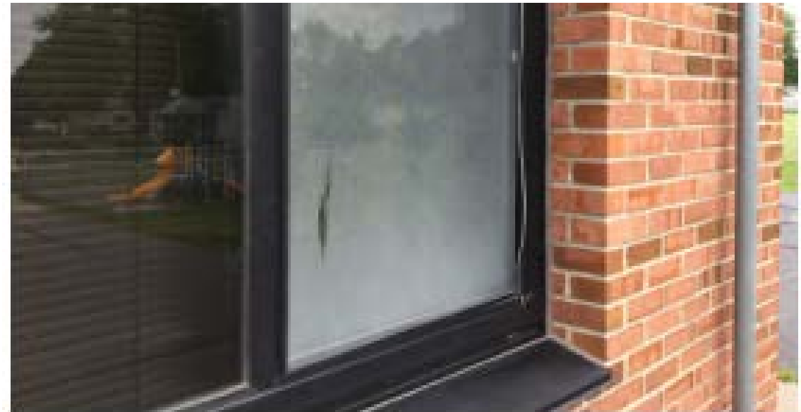
WINDOW REPLACEMENT (SINGLE PANE) ORIGINAL BUILDING
