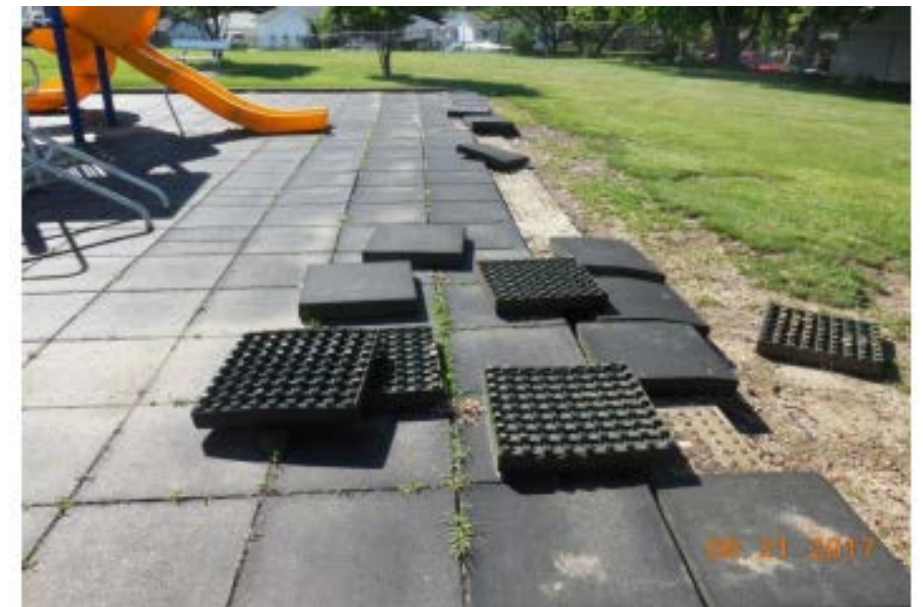
SITE DRAINAGE ISSUE WITH RUNOFF EROSION
