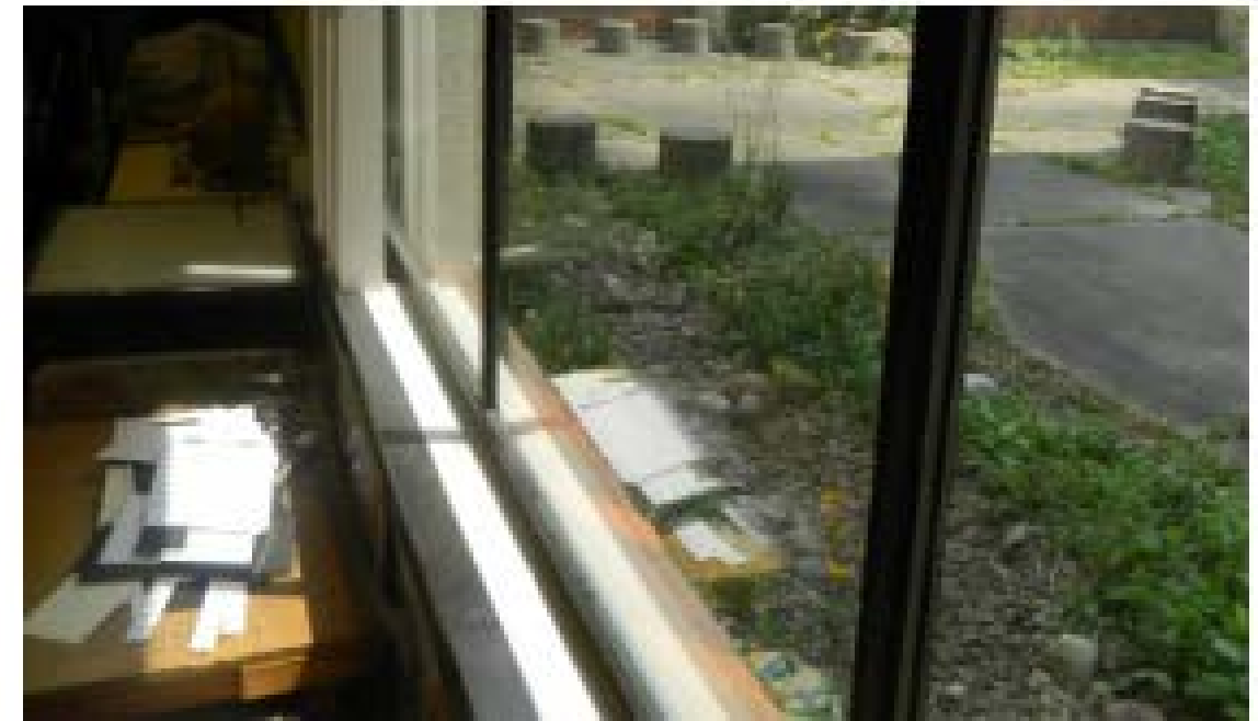
WINDOW REPLACEMENT (D100 & E100) NON-THERMALLY BROKEN FRAMES
