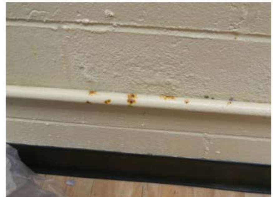
BASEMENT WATER INFILTRATION CONCERN
