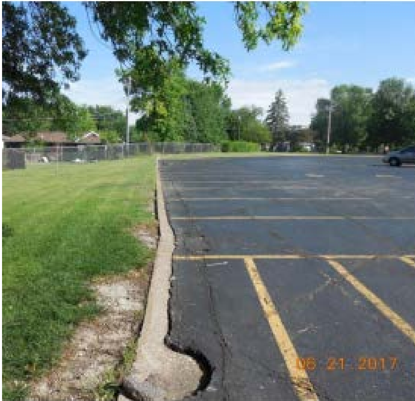
SITE DRAINAGE ISSUE WITH RUNOFF EROSION
