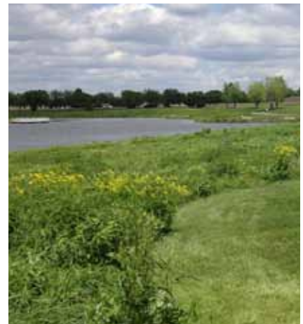
Above: A stormwater detention pond with a native vegetation buffer can manage stormwater and provide an amenity.
