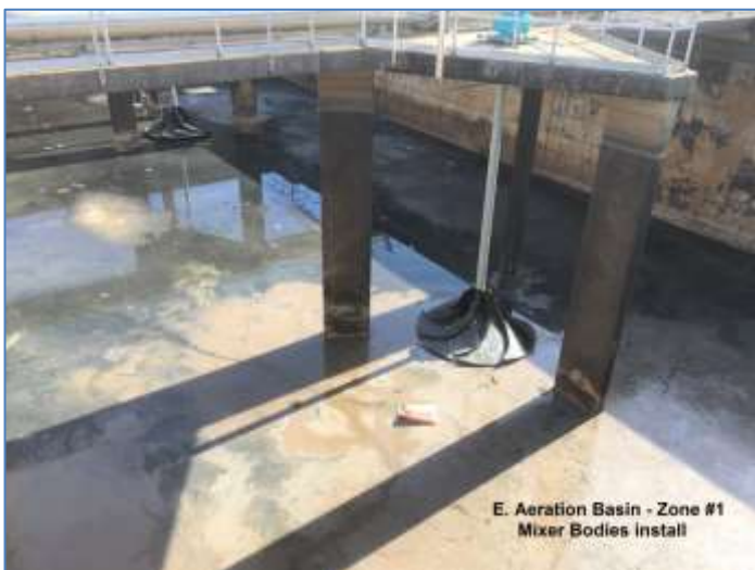
Aeration system – mixer installation
