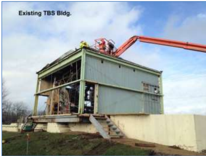
Demolition of existing TBS
