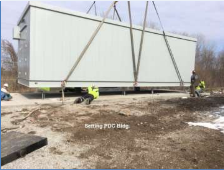
PDC building being installed
