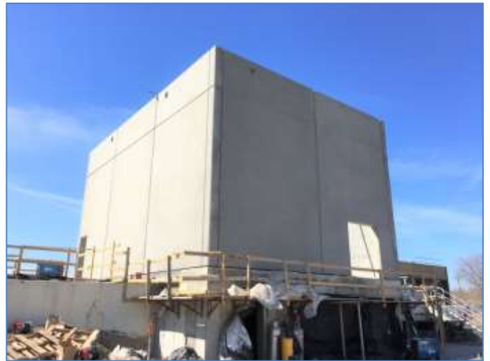
Construction of new TBS building
