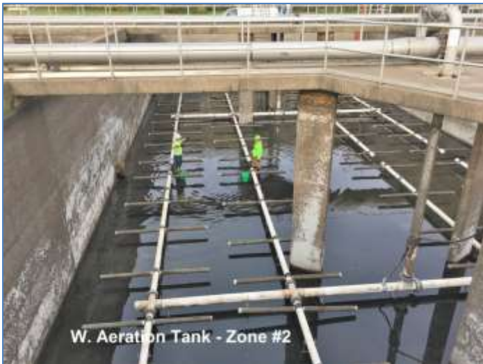
West aeration system improvements
