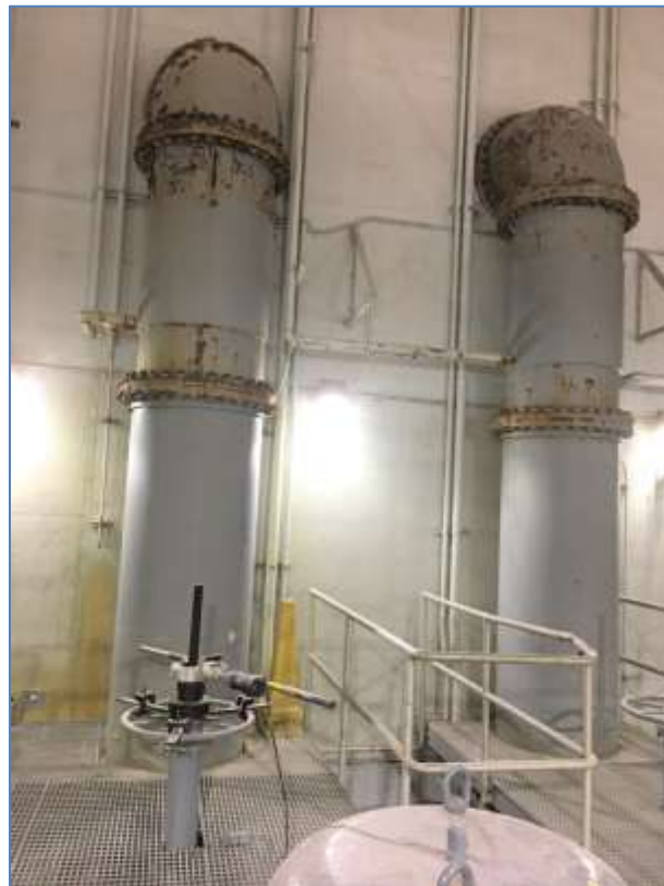
36" discharge pipes
