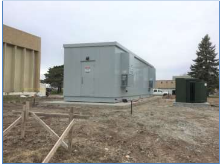
PDC installed on pad
