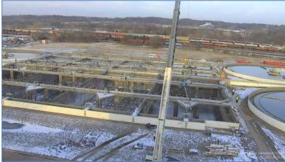
Aeration system improvements
