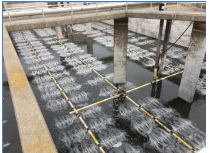
West aeration system improvements
