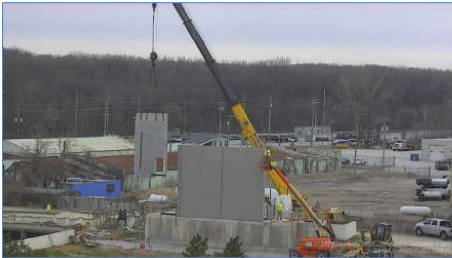
Construction of new TBS building
